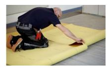
The required airing time depends on the temperature, the humidity and the absorbency of the sub-floor concerned. Therefore, it has to be ensured that the adhesive's open time is exceeded on no account. Make sure the adhesive has properly transferred to the back of the floor covering.
