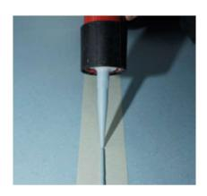
Immediately after application, the cold weld is pressed into the joint with the nora® smoothing spatula by running this evenly over the joint. Thereby, the surplus cold weld is pressed to the left and right of the joint. Hold the spatula in a position as flat as possible to avoid the development of hollow joints.
