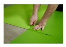
After the cutting of the seams/tiles fold back half of the sheets or turn over the rows of tiles. This method has the advantage of avoiding crooked joints or the shifting of joints because the tiles positioned on the floor serve as a stop for the tiles still to be installed.
