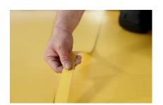
When installing norament<sup>®</sup>, experience has shown that it is best to cover the whole room or larger subdivided areas with loose tiles first, and then cut the border tiles, tiles for door openings, pipe apertures, etc. Thus, the tiles can adapt to the temperature of the subfloor.
