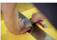
In practice we found it best to detach the half-cut strip with a hooked blade. We do not recommend cutting the underlying edge after embedding the floor covering as this implies the risk of the seam being compressed.
