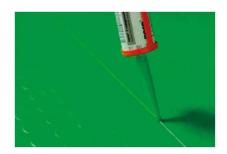
Immediately after application the cold weld is pressed into the joint with the nora® smoothing spatula by running this evenly over the joint. Thereby, the surplus cold weld is pressed to the left and right of the joint.
