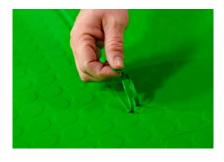
Even if no initial cleaning is required after installation, wax residues must be removed approx. 12 hours after joint sealing and at least 48 hours after installation with a suitable basic cleaner or oil and grease remover and a suitable method.
