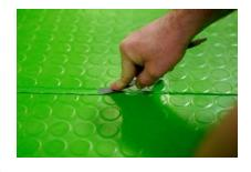
The surplus of cold weld pressed to the sides can be removed after approx. 12 hours.
