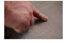
When the floor covering is embedded, it has to be ensured that the entire back of the floor covering is completely covered with adhesive. Position flooring edges without applying pressure. Under no circumstances should they be pressed or crushed. The breadth of the joints must not exceed 0.3 mm. Turn over the norament® tiles and place them accurately into the adhesive.
