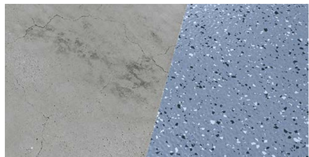
Installation with nora nTx on existing subfloors
