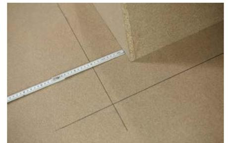
2. Position noraplan<sup>®</sup> and cut the seams. Apply adhesive exactly up to the marking and install the floor covering after airing.
