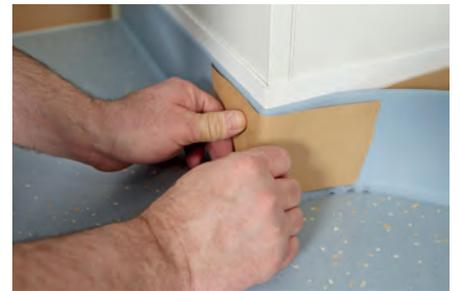
6. The **inside corners** are cut and butt-jointed.
