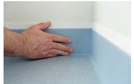
7. In order to avoid the formation of joints, the skirting has to be fixed at the corner with superglue.
