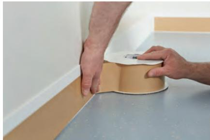
2. Clean the back of the skirting with a damp cloth - the back has to be residue-free.
