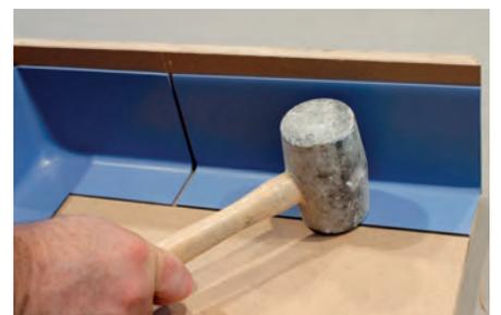
9. All joints along the skirting and skirting angles must be sealed with nora<sup>®</sup> 1 component cold weld. This can be done directly after the installation and the application of nora<sup>®</sup> liquid wax (see processing recommendation "Joint sealing").
