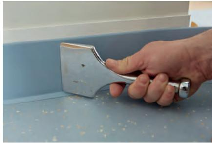
5. Heat the skirting for the **outer edges** with a welding gun and pull around the corner using slight tension.
