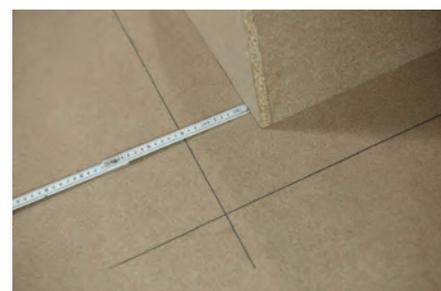
2. Position noraplan<sup>®</sup> and cut the seams. Apply adhesive exactly up to the marking and install the floor covering after airing.
