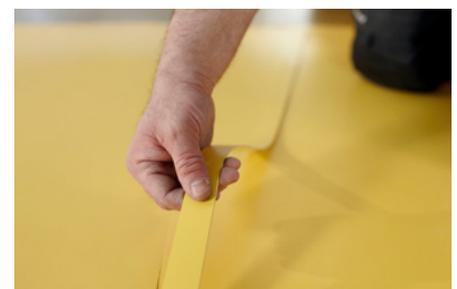
4. After seam cutting fold back half of the sheets.
