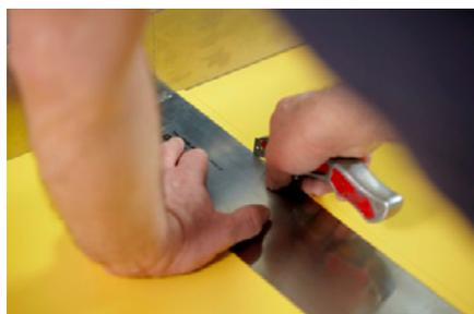
3. In practice we found it best to detach the half-cut strip with a hooked blade. We do not recommend cutting the underlying edge after embedding the floor covering as this implies the risk of the seam being compressed.
