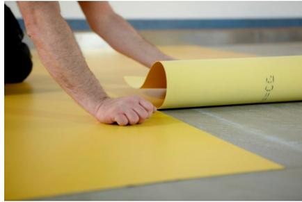
9. Carefully rub the floor covering on its entire surface into place, for instance with a cork board. Then press it down into position both longitudinally and transversely with a heavy iron roller (approx. 50 kg). When acrylic adhesives are used, repeat this procedure after a while (depending on the temperature), in particular at the ends and seams.
