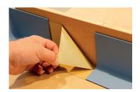
**8.** Then press the skirting and the skirting angles down and knock them into place with a light coloured rubber mallet.
