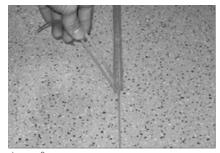
Inject the nora cold weld into the groove without gaps until a small bulb develops above the seam about the size of heat weld rod (Image 1). At the end of the seam, release the gun to prevent leaks. Any nora cold weld tracked or spilled on the flooring must be removed immediately using 70% Isopropyl alcohol and a clean cloth, cleaning at a later stage may not be possible.
