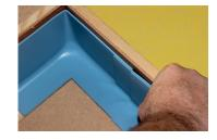
**6.** As the joints between skirting angles and skirtings have to be sealed, the skirting is placed in such a way to the angles as to create a joint width of 2-3 mm. Mark the skirting along the edge of this "ruler" using a straight blade.
