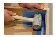
5. Next the skirting is cut. Between the inner and outer skirting angle the skirting requires a minimum length of 10 cm, shorten the angles if necessary. A piece of skirting is placed overlapping the affixed skirting angle. Use another stripe of skirting (minimum length 10 cm) as a ruler.
