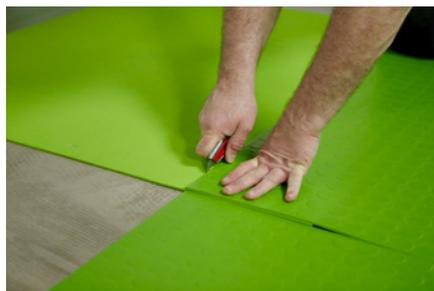
3. Then the rows of tiles are turned over and fixed. This method has the advantage of avoiding crooked joints or the shifting of joints because the tiles positioned on the floor serve as a stop for the tiles still to be installed.
