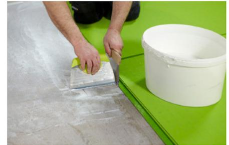
6. The required airing time depends on the temperature, the humidity and the absorbency of the subfloor concerned. Therefore it has to be ensured that the adhesive's open time is exceeded on no account. Make sure the adhesive has properly transferred to the back of the floor covering. Please observe additional information provided by the manufacturer.
