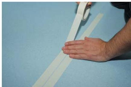
4. First seal the joints in one direction. After the cold weld has cured, seal the seams in the other direction. To do so, the 1-component cold weld is spread into the joints without leaving any gaps until a small bulge develops above the seam.
