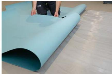
7. The required airing time depends on the temperature, the humidity and the absorbency of the subfloor concerned. Therefore it has to be ensured that the adhesive's open time is exceeded on no account. Make sure the adhesive has properly transferred to the back of the floor covering. Please observe additional information provided by the manufacturer.
