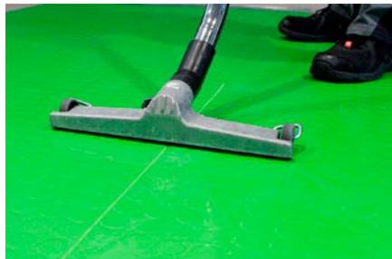
5. First seal the joints in one direction. After the cold weld has cured, seal the seams in the other direction. To do so the 1-component cold weld is spread into the joints without leaving any gaps until a small bulge develops above the seam.
