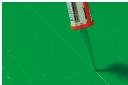
6. Immediately after application the cold weld is pressed into the joint with the nora<sup>®</sup> smoothing spatula by running this evenly over the joint. Thereby, the surplus cold weld is pressed to the left and right of the joint. You have to make sure that the cold weld pressed to the sides is entirely separated from the compound in the joints. Hold the spatula in a position as flat as possible to avoid the development of hollow joints.
