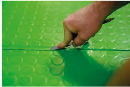
7. The surplus of cold weld pressed to the sides can be removed after approx. 12 hours.
