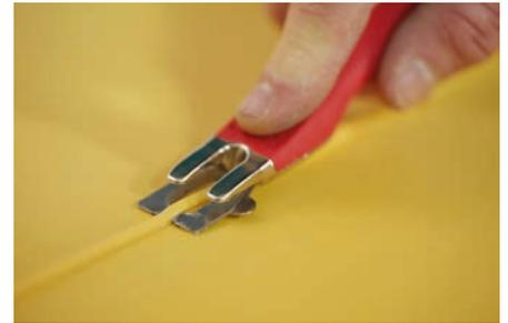
8. After cooling down the second cut is carried out with the Mozart knife without the distance sledge.
