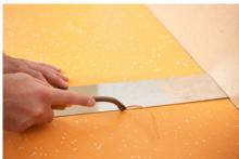
**2.** Joint width approx. 3.0 mm joint depth max. 1.5 mm
