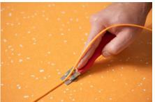
**8.** After cooling down the second cut is carried out with the Mozart knife without the distance sledge.
