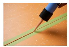
5. Immediately after application, the cold weld is pressed into the joint with the nora® smoothing spatula by running this evenly over the joint. Thereby, the surplus cold weld is pressed to the left and right of the joint. Hold the spatula in a position as flat as possible to avoid the development of hollow joints.
