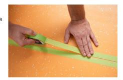
4. First seal the joints in one direction. After the cold weld has cured, seal the seams in the other direction. To do so, the 1-component cold weld is spread into the joints without leaving any gaps until a small bulge develops above the seam.
