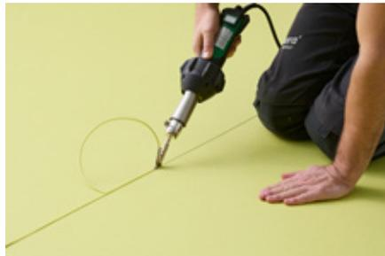
5. The processing temperature is 350-400° C (for noracare™ max. 300° C). Set the speed to approx. 2 m./min. The operating speed and temperature can be regulated on most welding machines.
