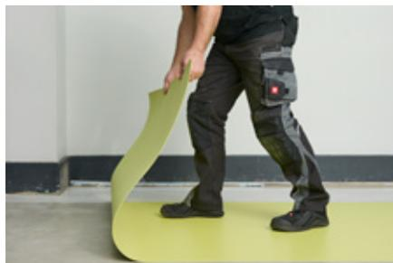
6. Cut and remove the protective paper of nora dryfix<sup>™</sup> 750, leaving an approx. 10 cm length from the flooring. Fold this 10 cm length underneath the flooring that has been folded back. This is meant to keep dirt particles away from the adhesive layer.
