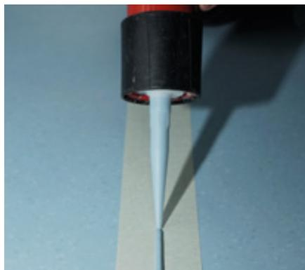
5. Immediately after application, the cold weld is pressed into the joint with the nora<sup>®</sup> smoothing spatula by running this evenly over the joint. Thereby, the surplus cold weld is pressed to the left and right of the joint. Hold the spatula in a position as flat as possible to avoid the development of hollow joints.
