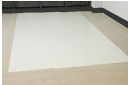
3. You can either trace-cut (using a ruler as a guide) or double-cut the seam between two nora dryfix™ ed strips. Take care not to leave any gaps wider than 2 mm.
