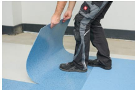
6. Cut and remove the protective paper of nora dryfix<sup>™</sup> ed, leaving an approx. 10 cm length from the flooring. Fold this 10 cm length underneath the flooring that has been folded back. This is meant to keep dirt particles away from the adhesive layer. In case nora dryfix<sup>™</sup> ed is cut through, please connect both parts with a copper strip.
