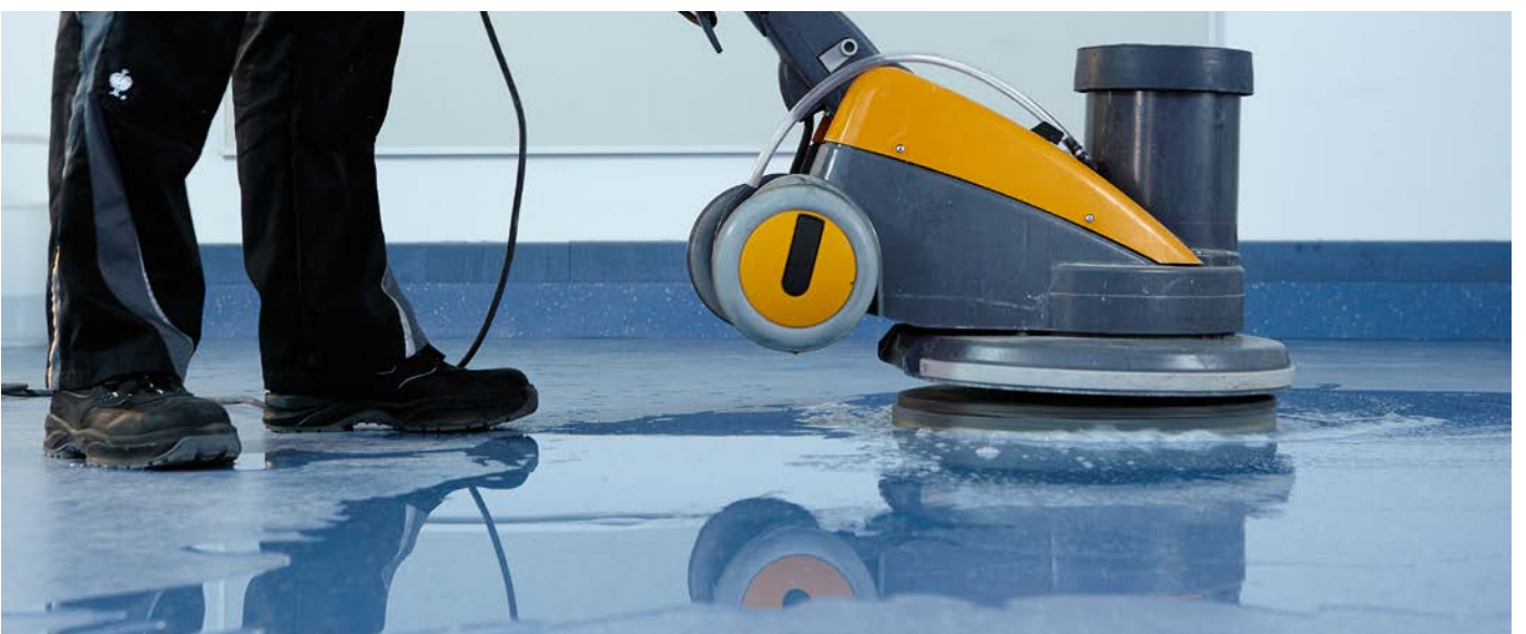
Refurbishment. Removing the most stubborn dirt and scratches
