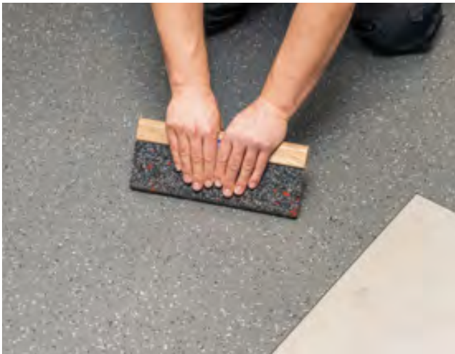
Rub the floor covering with a cork board
