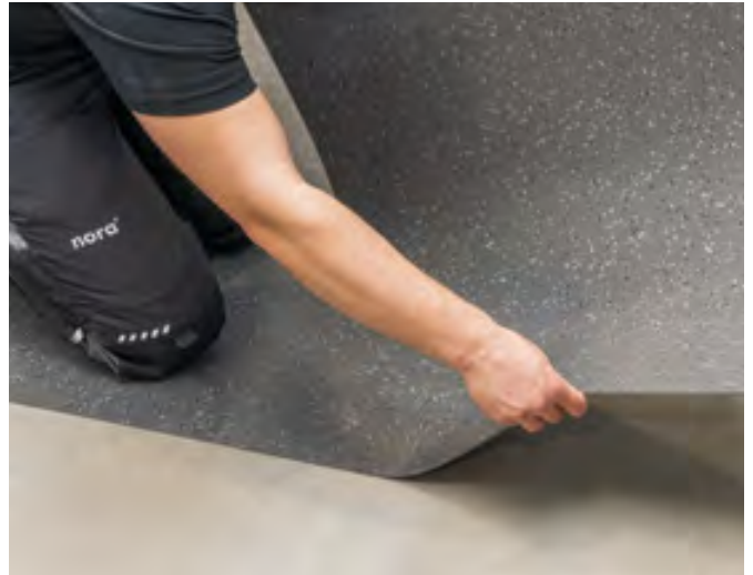
Install the floor covering
