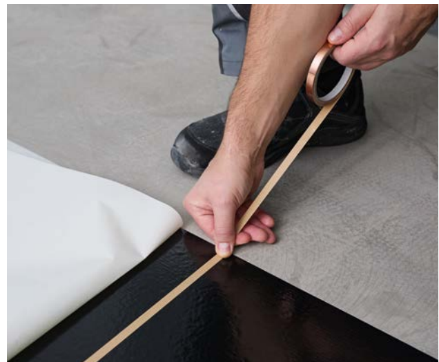
Bond the copper strip
