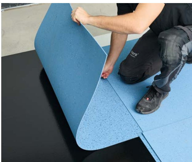
Install the floor covering
