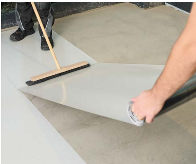
Lay nora dryfix ed on the subfloor
