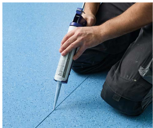
Seal the floor covering
