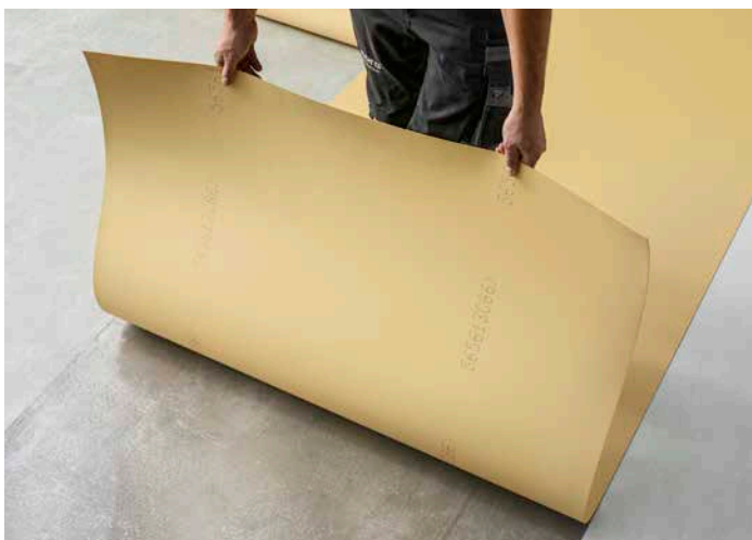
3) Install the floor covering
