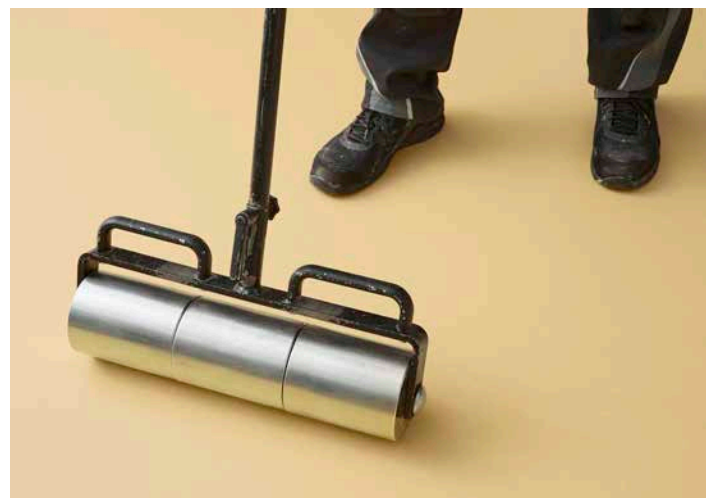
4) Roll the floor covering and weld where specified
