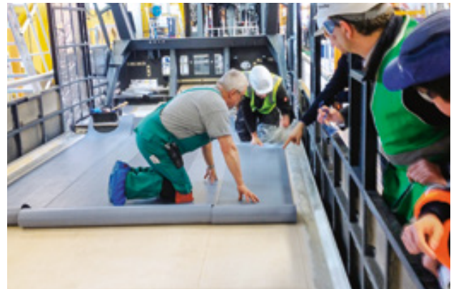
Ongoing nora nTx installation
