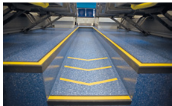
Stair nosing with signal stripes
